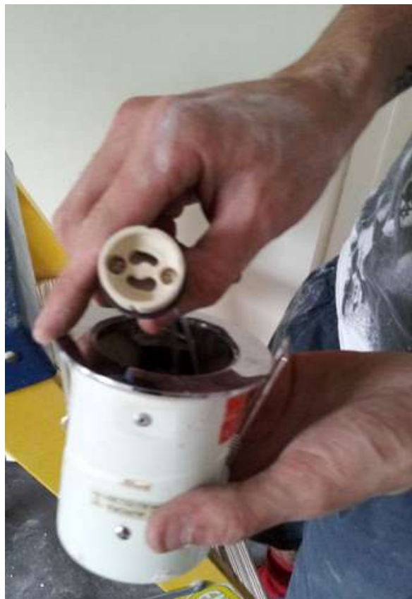
Fig.3 Downlighter converted to GU10
